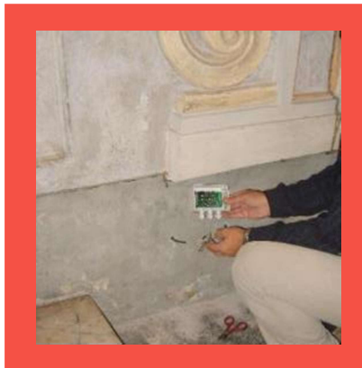
sensor probes installation
